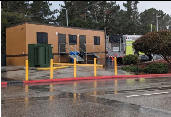
Modular trailer "fire station" at airport
