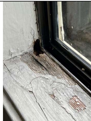
Kitchen area windowsill
