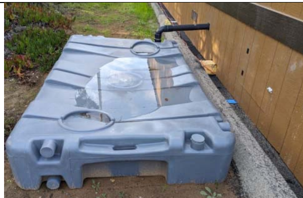
Septic system for modular trailer
