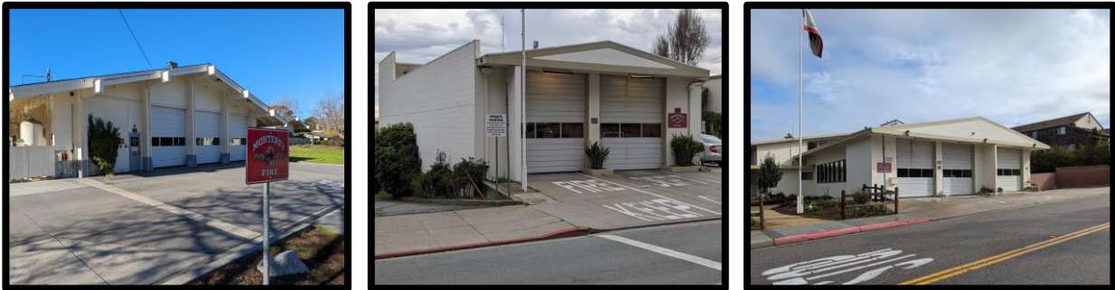
From Left: #11 Pacific Street, #12 Hawthorne Street, and #13 Del La Vina Source: Photograph taken by Civil Grand Juror
